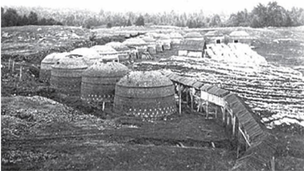
Fig. 1.6: Brick laid beehive charcoal kilns near the Katahdin Ironworks (ca. 1843 to 1890) similar to the design and layout of the ones used for the Woodstock Charcoal and Iron Company (ca. 1848 to 1889) (Maine Geological Survey, 2005).
